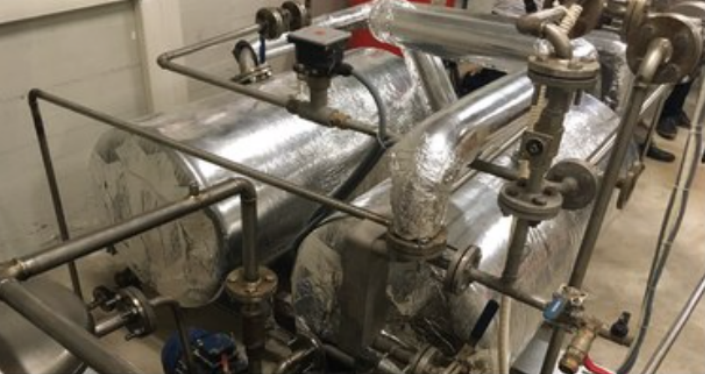
Testing ZERO BRINE technologies at the Brine Excellence Center at National Technical University of Athens
