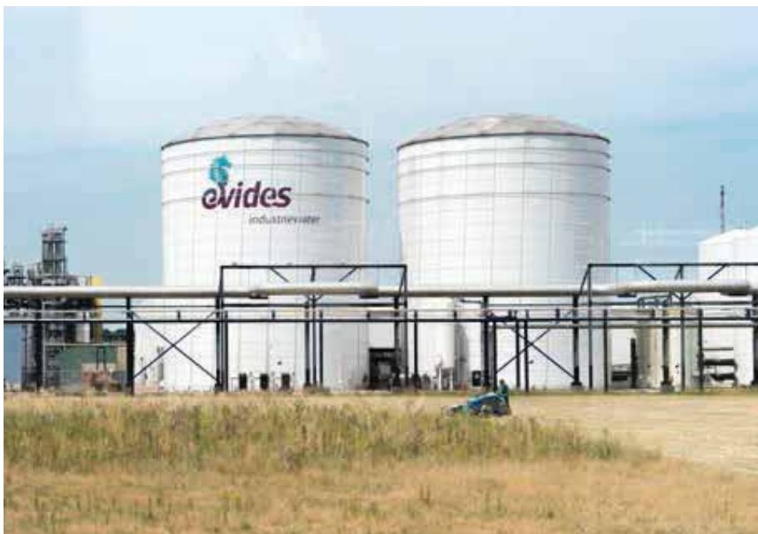
Above: View of the Evides Industriewater demineralized water plant, located at the Botlek industrial area at the Port of Rotterdam.
