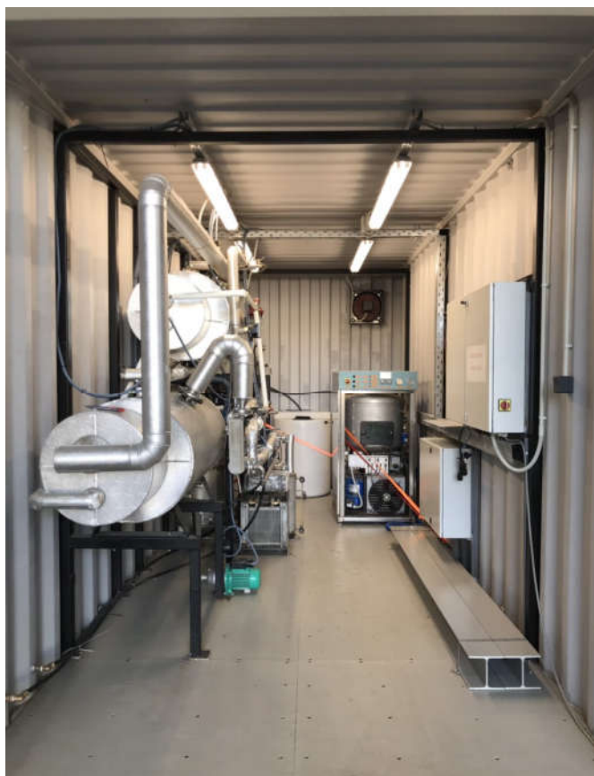
Installation of the MED-NTUA Evaporator & of the Crystallizer (March 2019)
