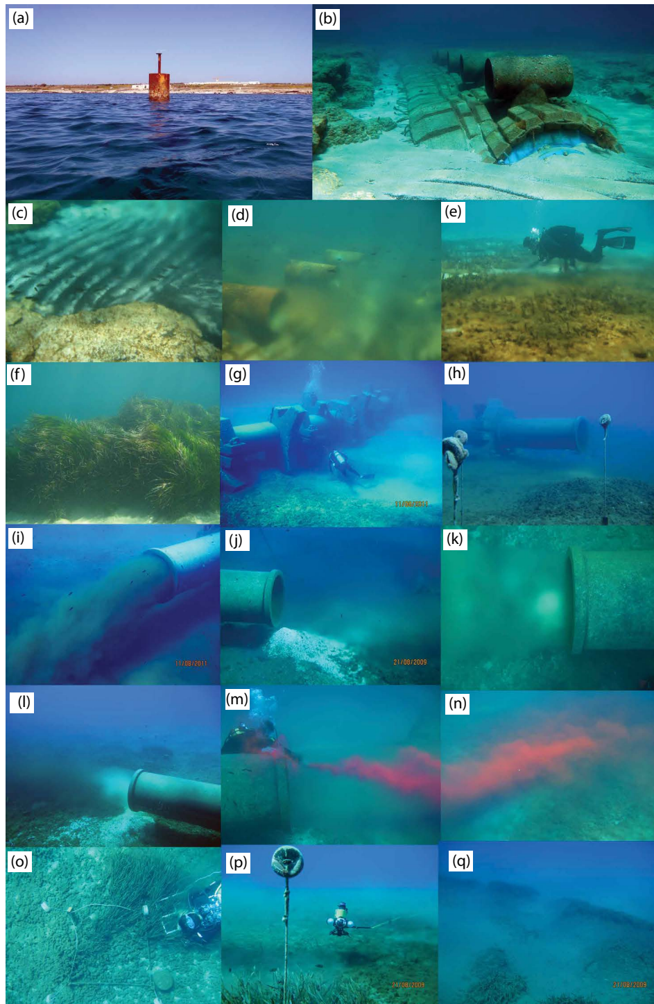
Fig. 1. In situ photographs of the desalination plant outfalls at Dhekelia and Larnaca. (a–f) Dhekelia. (a) Surface marker buoy of the outfall. (b) Overview of the outfall structure. The brine outfall pipe is covered by concrete padded-mats such as those used in the offshore oil and gas industry, with orthogonal, multidiffuser pipes standing above it. When this photo was taken, no brine was being discharged. (c) Due to the marked difference in density, the brine tends to sink into local depressions, causing turbid conditions. (d) The diffuser pipes discharging brine. (e) Diving survey of the vicinity of the diffuser pipes. Note the brine collecting near the seabed, visible by the turbid layer beneath the diver. (f) Posidonia oceanica meadow near the outfall pipe. (g–q) Larnaca. (g) Overall view of the outfall pipeline. (h–k) The brine outfall at different levels of plant operation: inactive (h), full operation (i), and intermediate levels (j–l). The outfall also contains insoluble solids, which precipitate at the outfall pipeline (j). In order to trace brine dispersion, a diver injected rhodamine, a fluorescent dye, into the outfall (m,n). Posidonia meadow health is monitored in long-term quadrats deployed on the seabed (o). Diving surveys are further supported by remotely operated vehicle (p). Near the outfall, brine impacts on seagrass are clearly visible (q).
