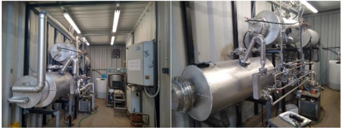
Figure 15: MED EVAPORATOR REFURBISHED AND CONTAINERIZED
