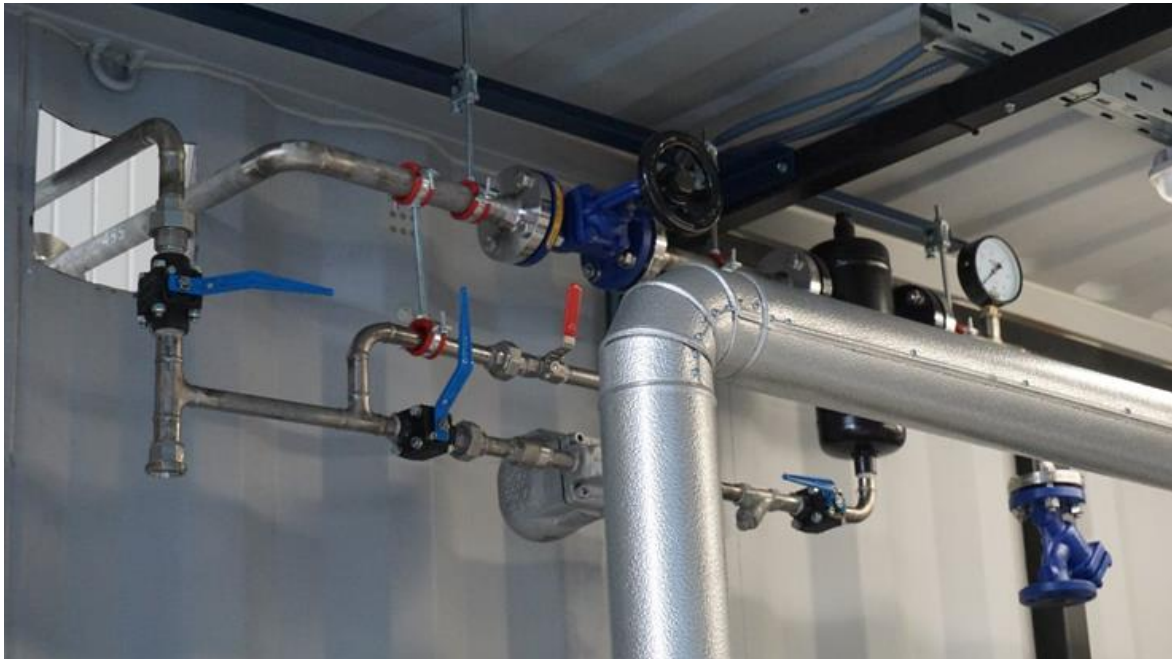
Figure 12: INSTALLED EQUIPMENT FOR RESIDUAL HEAT USE IN MED EVAPORATOR.
