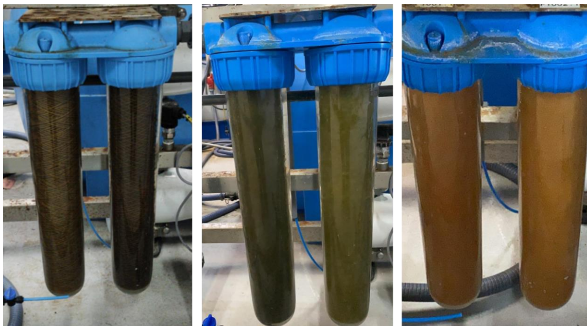
Figure 50: CARTRIDGE FILTERS OF THE NF UNIT ON 12 OCTOBER 2020 (LEFT), 18 NOVEMBER 2020 (MIDDLE) and 19 MARCH 2021 (RIGHT)
